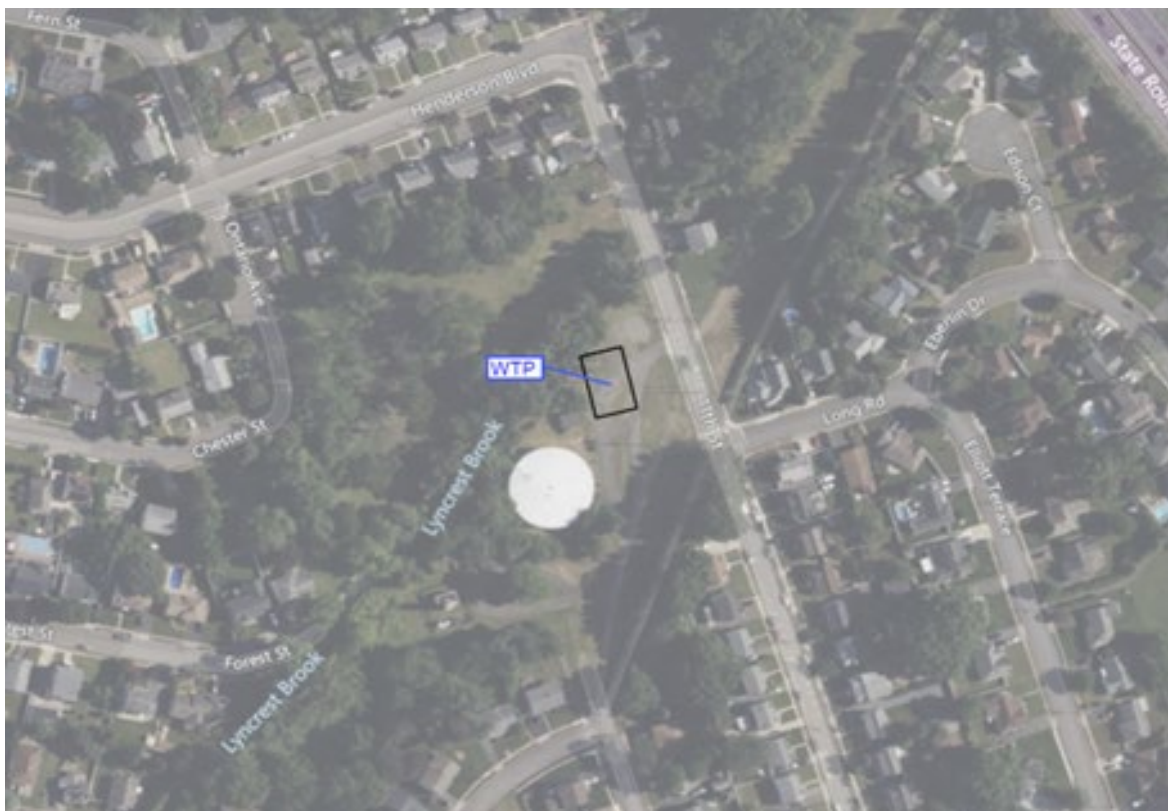
Location of the new groundwater treatment facility along 11 th Street in Fair Lawn, New Jersey. Shown here as a blue rectangle.
